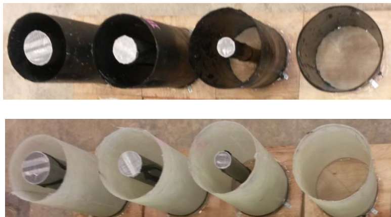
Figure 1: Ready for concrete pouring of FSDTs and CFFTs
